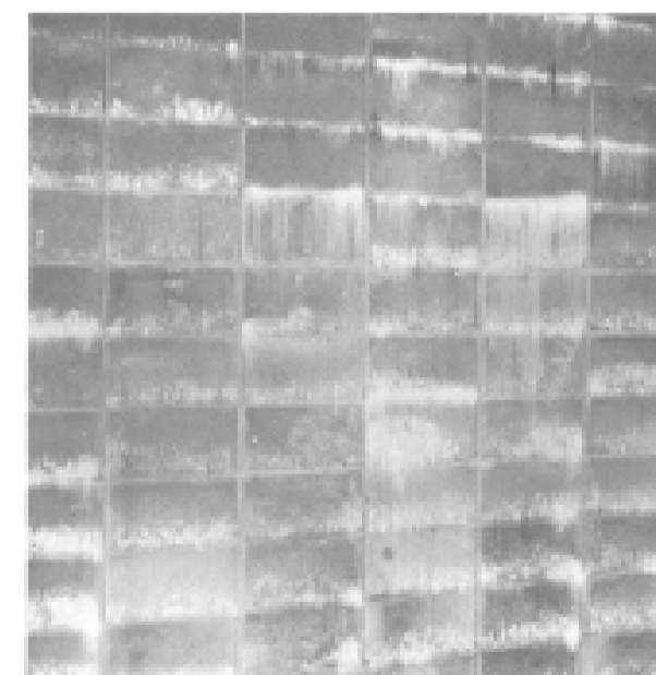
Fig. 1. Photo of masonry wall.
