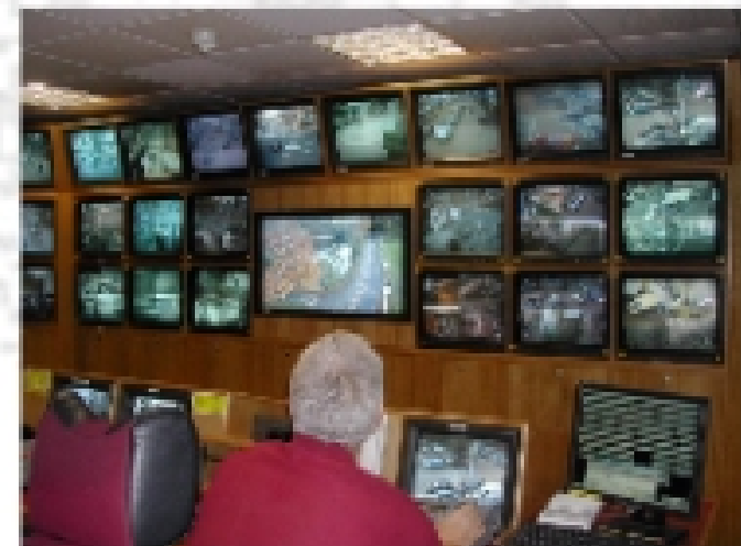
Law Enforcement: CCTV control
