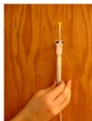
Use a depth gauge to determine where the spinner should be.
